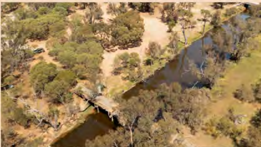
Pumphreys Bridge. Image by Andrew McKenzie
