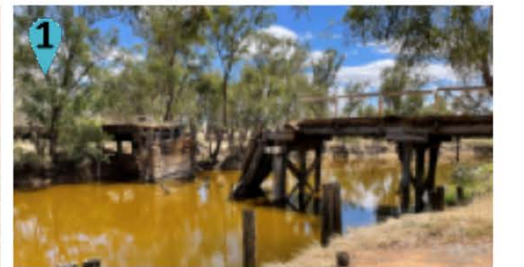
1 Remnants of the old bridge-deck have been left hanging in the river channel and may be unsafe. A structural inspection is recommended to determine how much of the structure can be retained and repurposed (see note 11).
